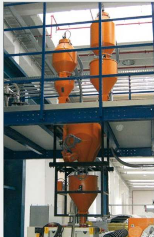
Graviko type GK 1000 (with a loss-in-weight control system)
